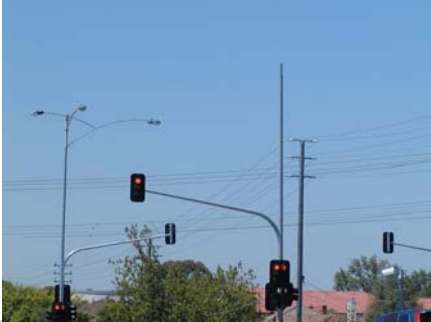
A Recently Remodelled Intersection Where Lighting Has Not Yet Been Installed
